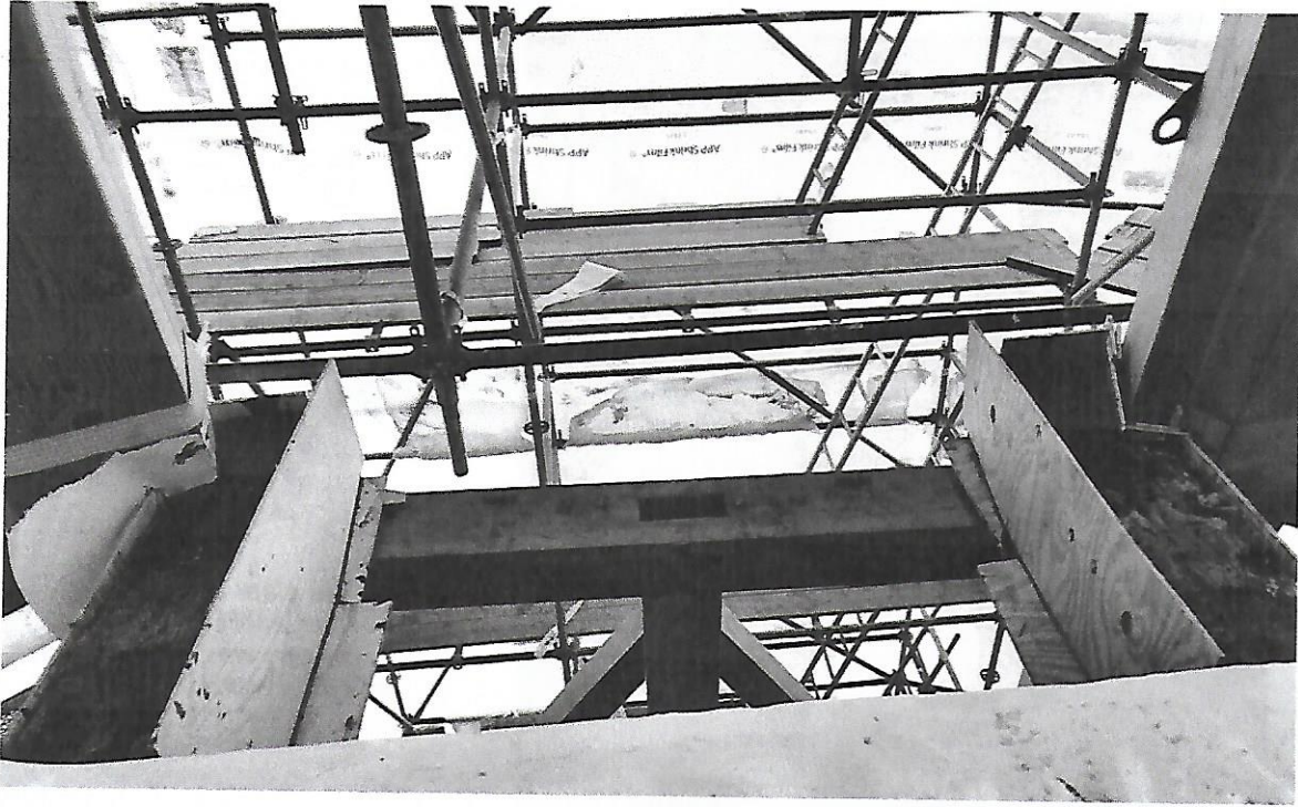
6. This photo shows shuttering in place following the repair of two of the beam ends.
