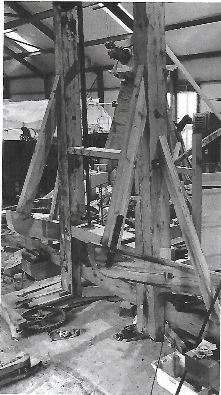
13. A detail view of the fantail frame assembly. Much of the existing timber has been retained and the side braces have been replaced at the correct angle. The re-machined down shaft is back in position.
